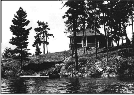
Second Cache Bay cabin on the southeast point of Cache Bay. The cabin was built in 1938. It was a very exposed location for aircraft landings so the next and present cabin was built on an island in Cache Bay in the 1950's. [Lloyd Raven collection].
